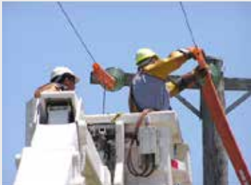
Live line work (elevated electric fields also)
