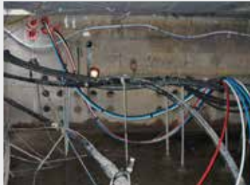
Cable pits and basements
