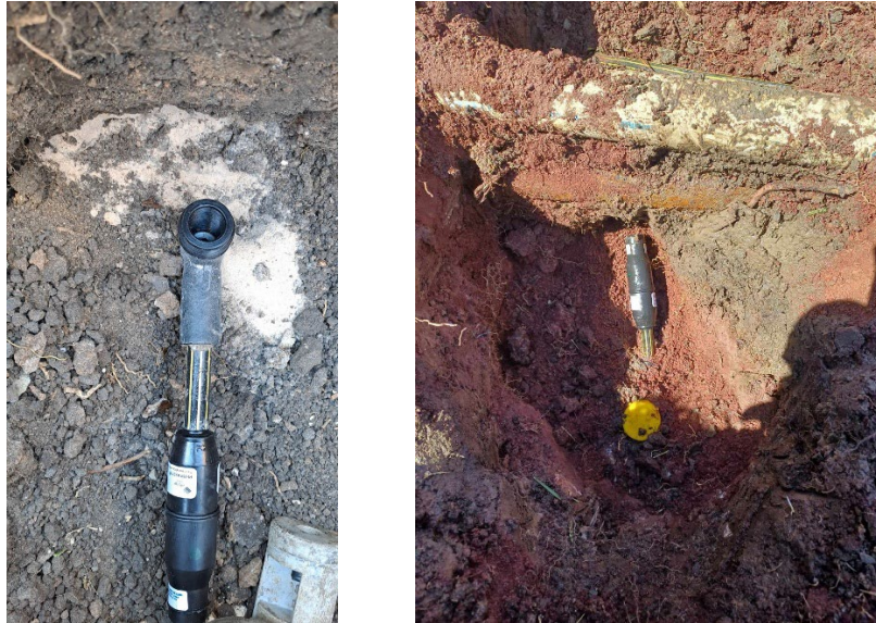
Figure 1 Example -Service tapping saddle with cutter wound down, and service pipe capped.
